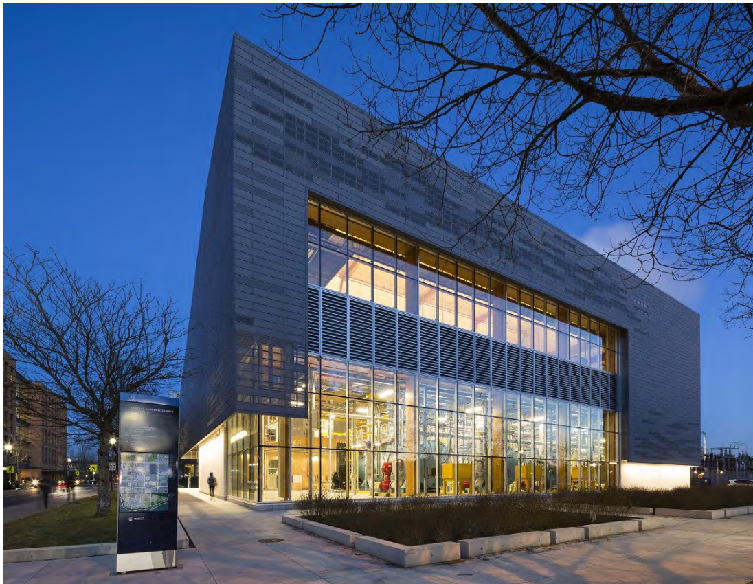
Figure 11: UBC Campus Energy Centre 8
