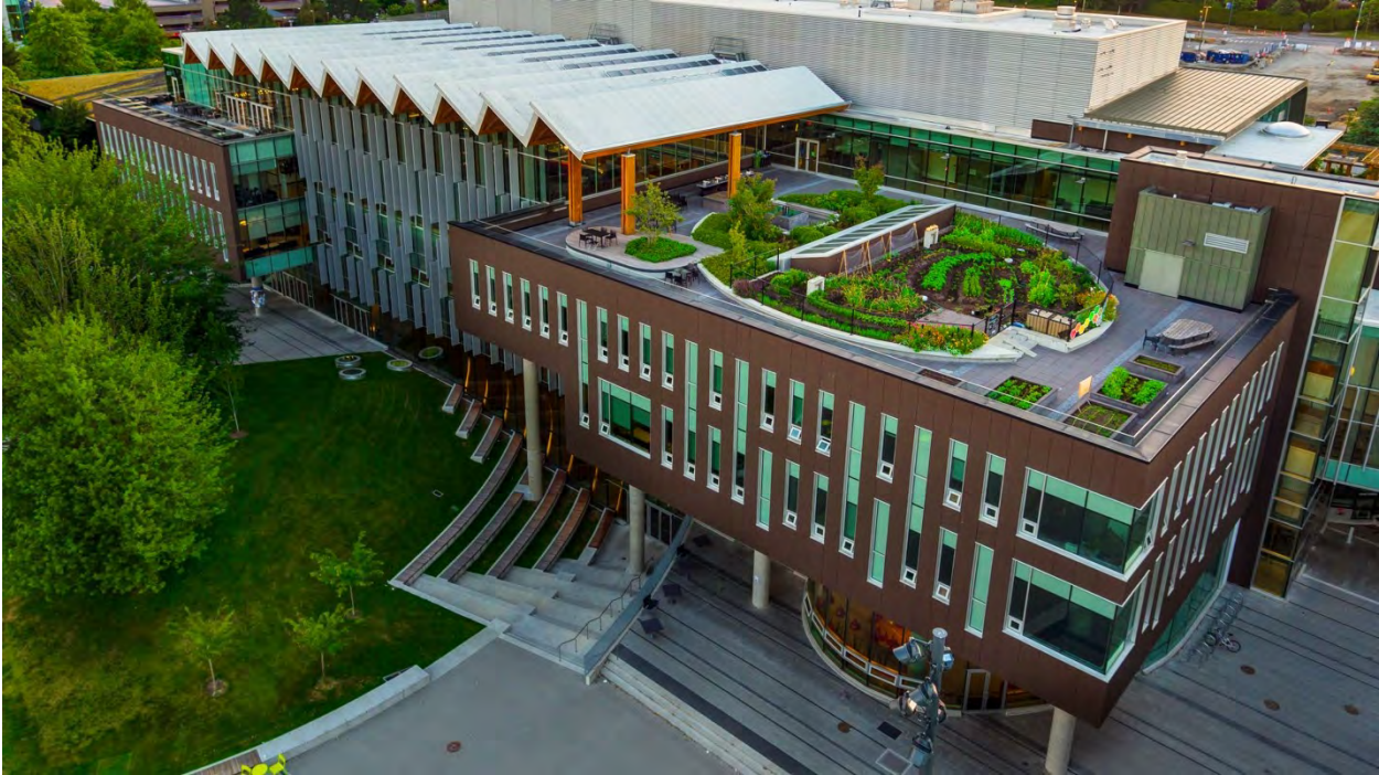
Figure 13: UBC Nest Building with roof top garden
